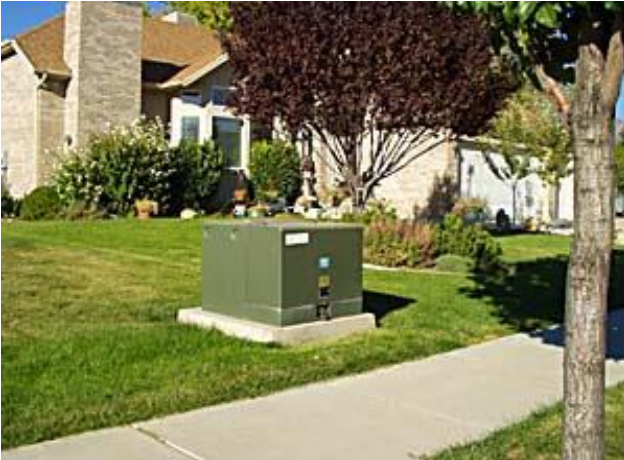
Figure 1A: Pad-mounted Equipment (Underground System)
